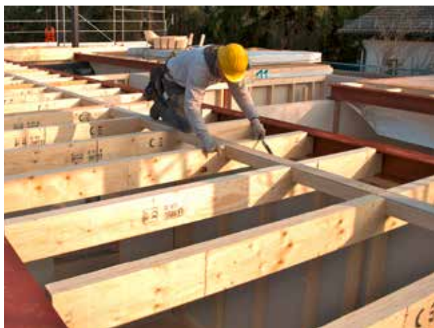
STEICO LVL R used for the construction of high load bearing floor structures
